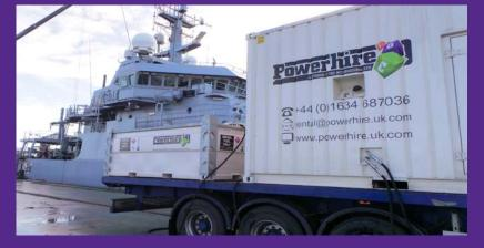
power rental equipment at their Kent site and delivered it to Falmouth. Once onsite the engineers set up a 1000kVA generator and 6,000Ltrs fuel tanks together with 100metre 240mm 3 phase cable connecting it to the Royal Navy Vessel. Before leaving site Powerhire engineers commissioned the power hire package to ensure it's effectiveness for the duration of the three week hire period.
