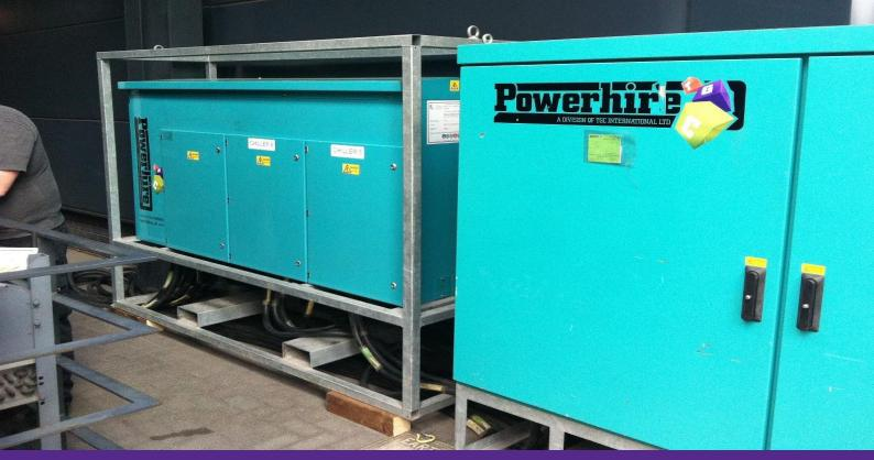
Two smaller MDU's were set up at ground level at the end of a walkway and supplied by substation 3 with connection to the 2 remaining temporary chillers.
