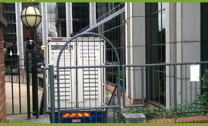
Our Technical Sales Manager specified one of Powerhire's super silent enclosed 1000kVA generators to act as the site's temporary back-up generator power. This would function in the exact same way as their current system had previously performed and be called into action should there be any loss of mains power. This would also enable the installation of the new permanent backup generator system at the site.
