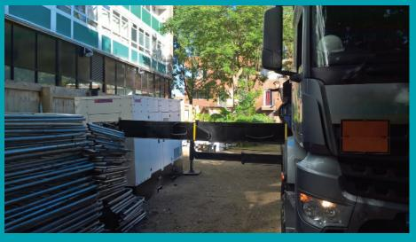
x 300kVA silenced generators in N+1 mode being delivered and installed, meaning that in the event of a fault, Generator 2 would instantly be called for to take up the load. During the hire period, Generator no. 1 ran faultlessly, so generator no. 2 was not called for.
