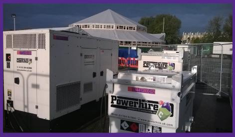
of our modern and fuel efficient 100kVA prime rated Bruno generators, a 2000 litre fuel tank along with an additional 950 litre road tow fuel bowser to cover the unlimited running of the generator.
