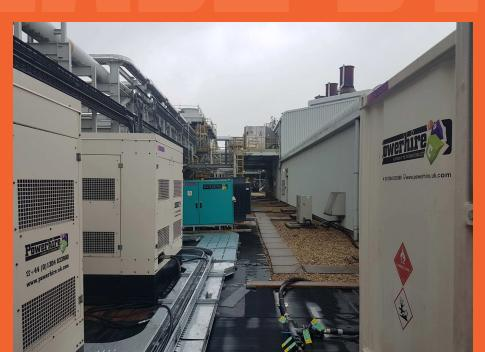
A separate order was then placed for a 4th 500kVA generator set to be installed on the site to act as an emergency standby generator for essential services at another part of the site.
