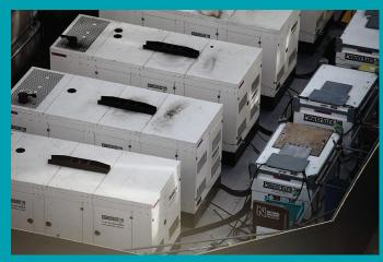
It was requested by the client that the temporary power be located in the courtyard of the museum but later in the design stage it was determined that owing to loss of car parking spaces and the proximity of the generators to the switchroom the equipment would be located on the grassed areas either side of the accessible road leading to the courtyard and adjacent to the building where the switchgear is situated.
