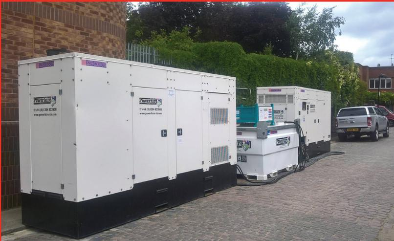
Powerhire were contacted by the project director of Sparq with regards to the hire of temporary generator power to support their equipment being utilised for this amazing event. The customer knew the exact size generators that were required and requested 2 off 200kVA Silenced Rental Generator SYNC sets, both running together in sync, so if one fails the other will seamlessly continue to provide power, and 1 off 3000 Litre Bulk Fuel Tank.
